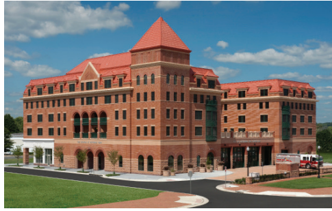
City of Alexandria, VA, Fire Station 209 – Station at Potomac Yard.
