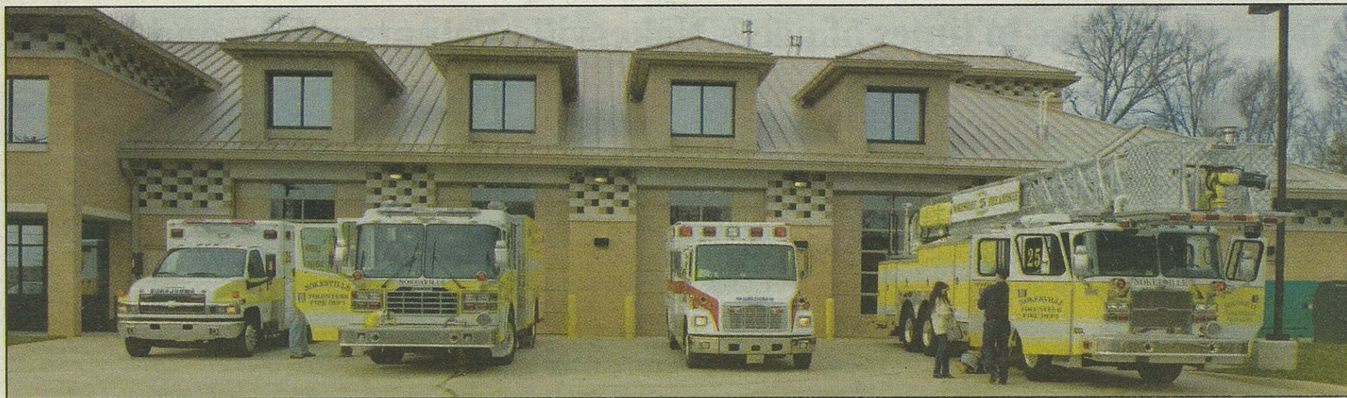
Emergency vehicles in front of the new Nokesville Volunteer Fire and Rescue Department station 25.
