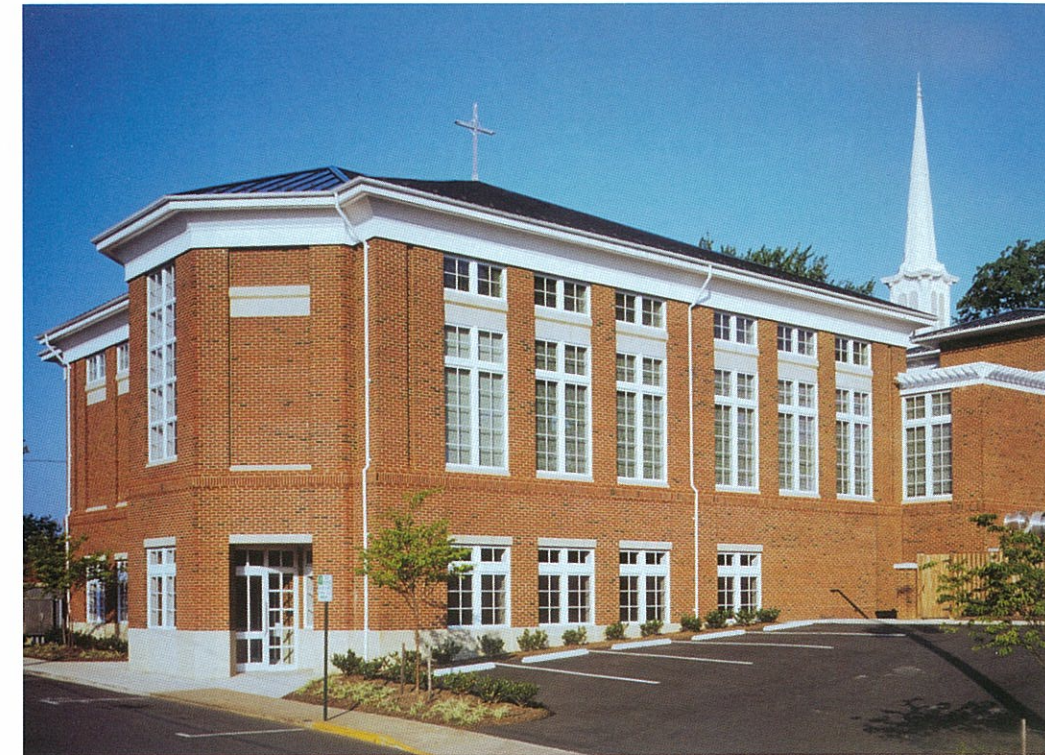
A parking lot located on the south façade allows room for future expansion of the sanctuary on the upper level and the fellowship hall below.
